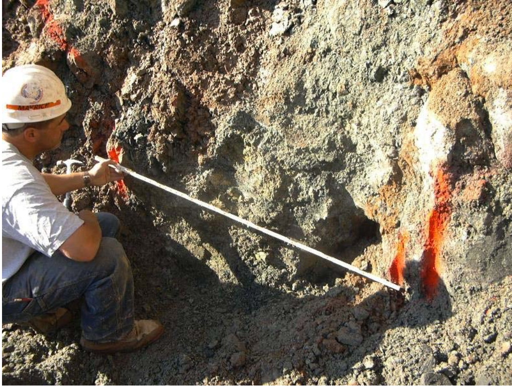
Photo 6 – Weathered Rock Below Sheeting
