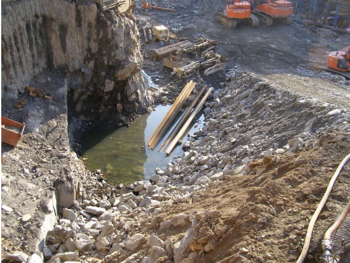
Photo 10 – Face of Rock after Blasting on 7/25/07
