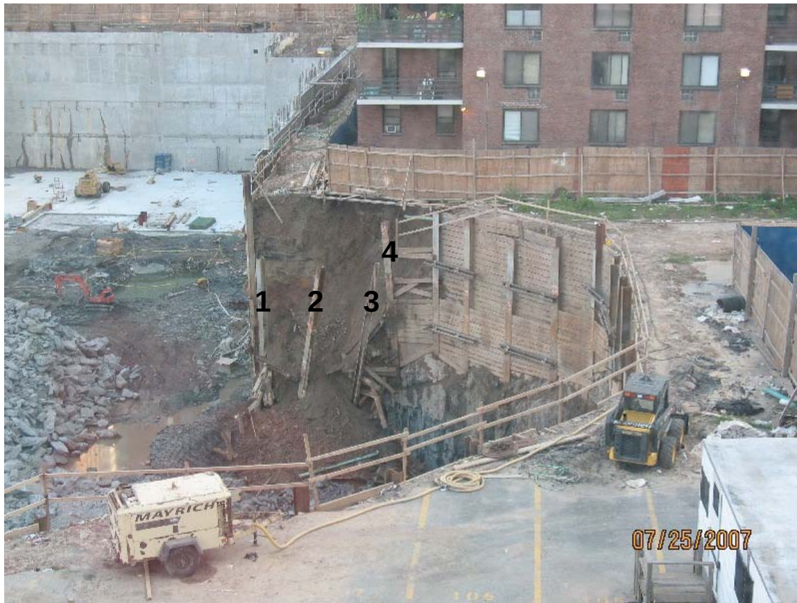
Photo 5 – Collapsed Sheeting
