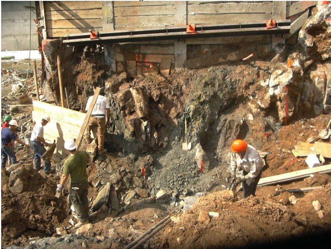
Photo 7 New Sheeting Installed Several Feet Away From Original. Note Weathered Condition of Rock
