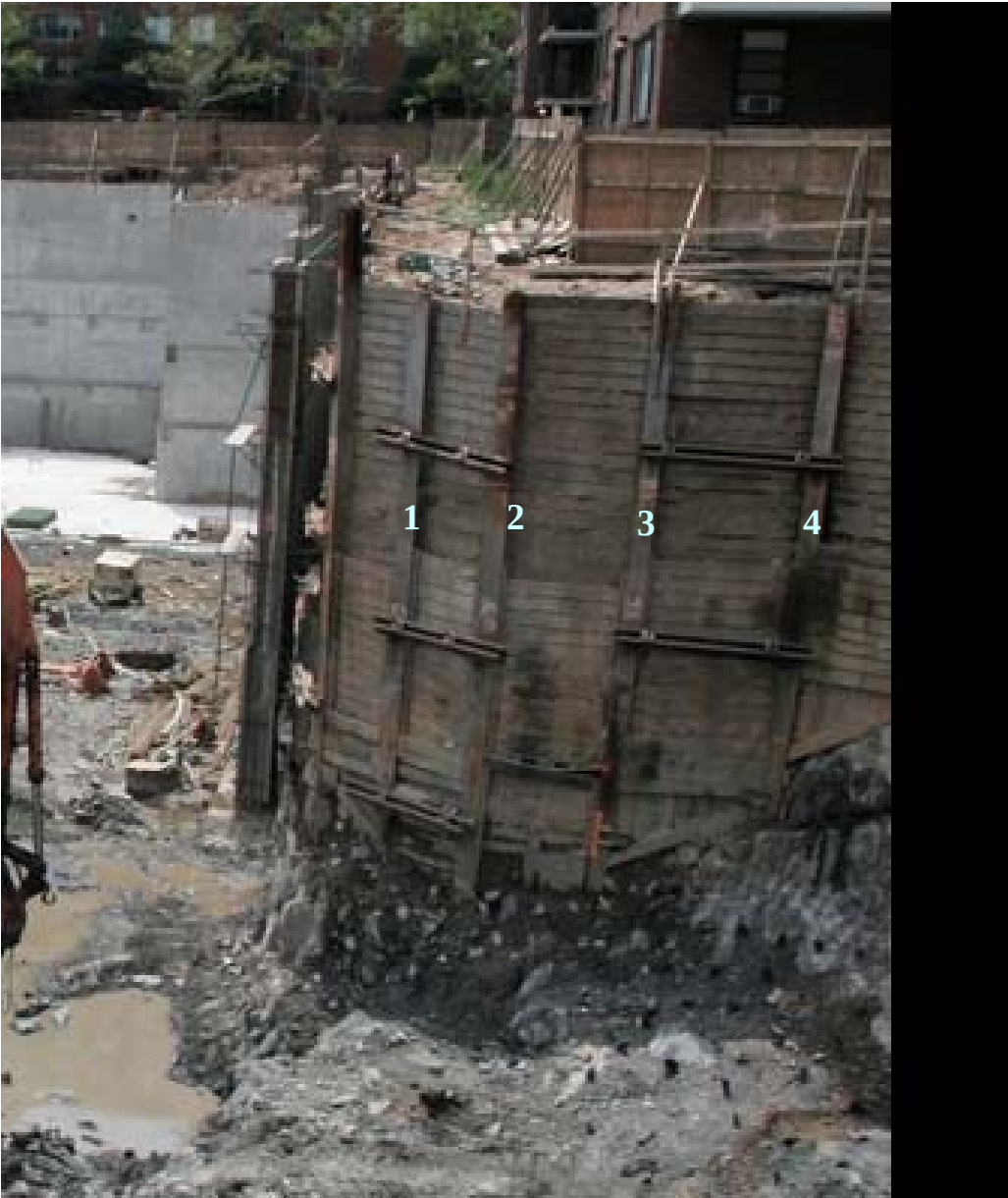
Photo 4 – The Sheetting Wall Pre-Collapse –Bernstein photo 7/20/2007
